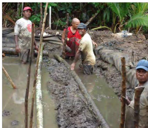
An adaptation project in Palau: Construction of a dike system in a taro patch to reduce the impacts of sea level rise, coastal erosion, flooding, and salt water intrusion © PCC.
